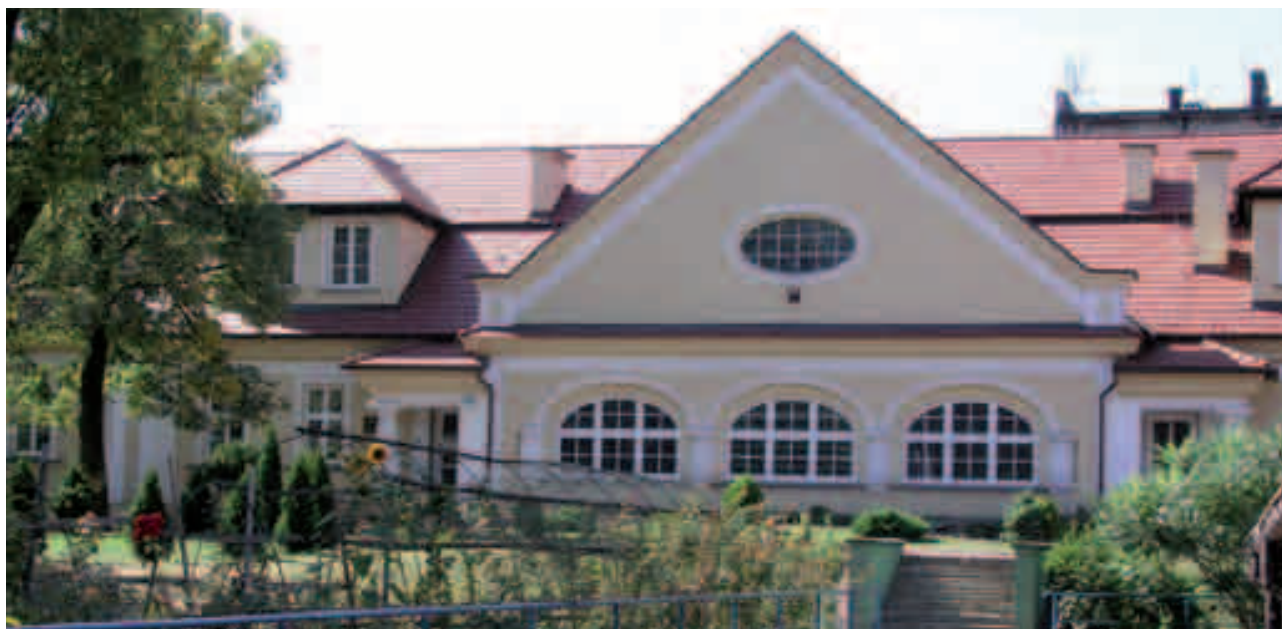
W dawnym Domu Kawalerów osiedlił się Zakon Misjonarzy z Marianhill./ The Order of Missionary's from Marianhill has settled the old House of Cavalier's.
